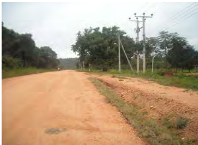
Date : Feb. 16, 2010 Place: Moragahakanda Dam Site Title: Diversion road with 33kV power transmission line
