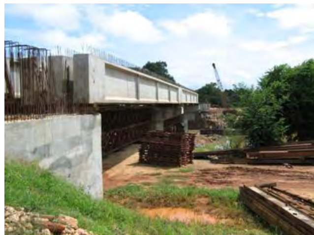
Date : Feb. 2, 2010 Place: Moragahakanda Dam Site Title: Amban Ganga Bridge
