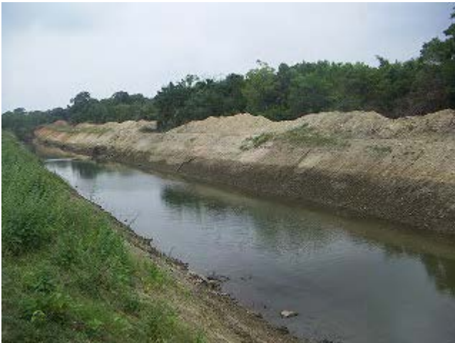
Date : Feb. 3, 2010 Place: Kaudulla Left Bank Title: Improvement Work of Kaudulla Left Bank Main Canal (Existing: 6m – New: 9m)
