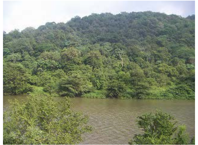
Date : Feb. 2, 2010 Place: Moragahakanda Dam Site Title: Dam Axis of Main Dam, view from left bank
