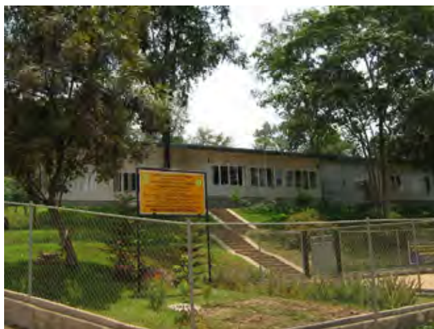
Date : Feb. 2, 2010 Place: Moragahakanda Dam Site Title: Moragahakanda Project Office
