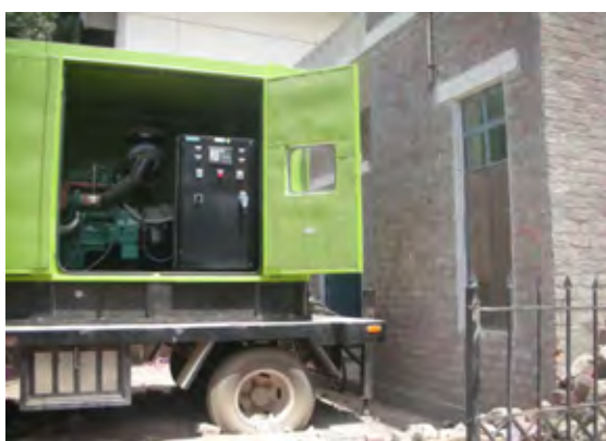
Tube-well with Generators (200KVA)
