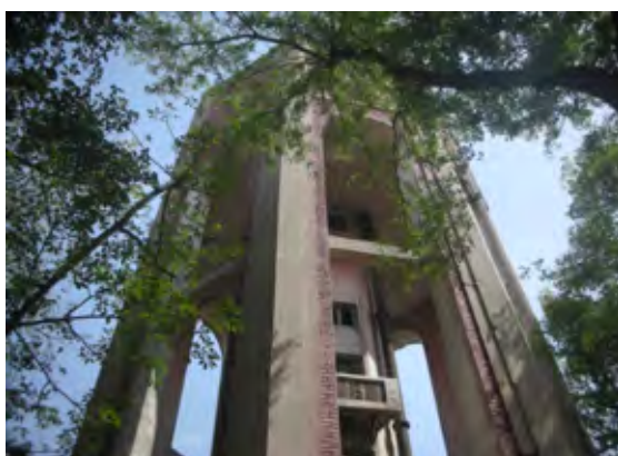
Abandoned Elevated Tank (60,000gallons cap.)
