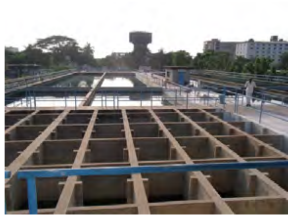
[Baffling type flocculation basin and sedimentation tank in Godnail Purification Plant of Dhaka WASA] The plant is along with Shitalakshya River for water intake.
