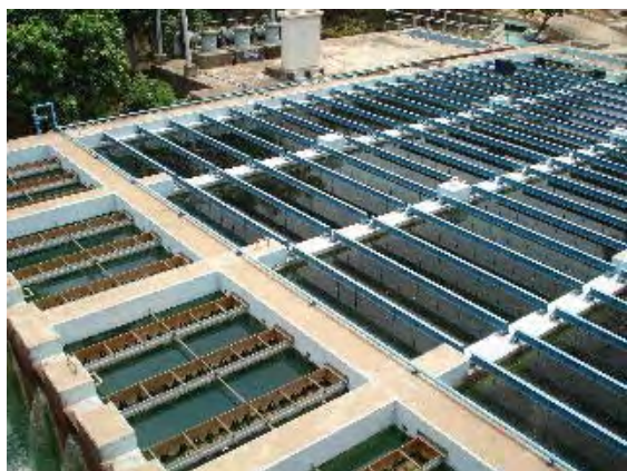
Figure3.13-3 Baffle Plate Sedimentation Pond in Chandnighat Plant
