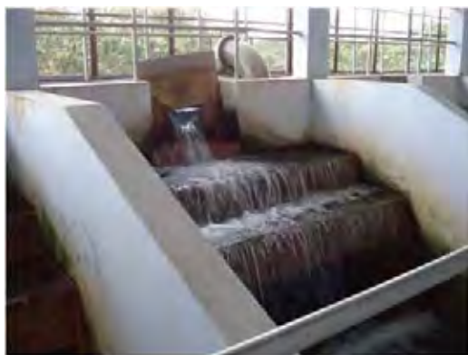
Figure 3.13-6 Iron Removal Facility in Noakhali (Oxidation Ditch)
