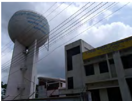
[Elevated water tank in Noakhali] The tower is in the site of iron removal facility. It is also used for backwash of filtration pond.
