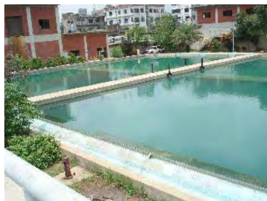
Figure3.13-2 Sedimentation Pond in Chandnighat Plant
