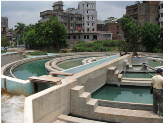
[Rapid mixing tank and slow mixing tank in Chandnigahd Purification Plant of Dhaka WASA] Flock formation by water flow is satisfactory.
