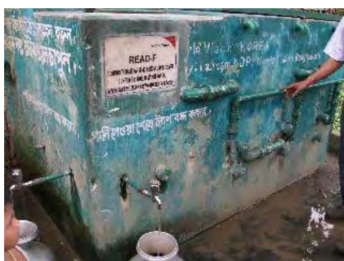
Figure 3.12-2 “READ-F” (which is one of arsenic removal equipment for community use)
