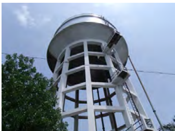
[Elevated water tank in Brahmanbaria] Groundwater from a well is delivered through this tower.
