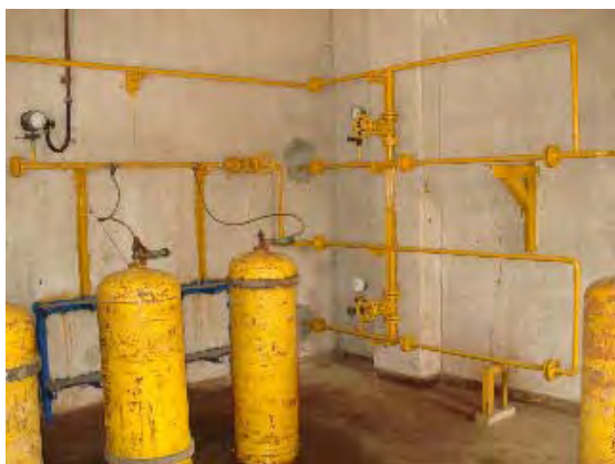
Figure3.13-4 Steel Cylinder Bottles of Chlorine in Chandnighat Plant
