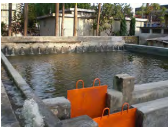
[Sedimentation pond in Khulna WASA] Filtration pond is broken and sedimentation treatment water is distributed.
