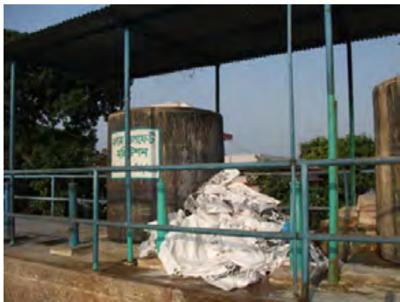
[Aluminum sulfate facility in Godnail Purification Plant of Dhaka WASA] Solid aluminum sulfate is used as coagulant.
