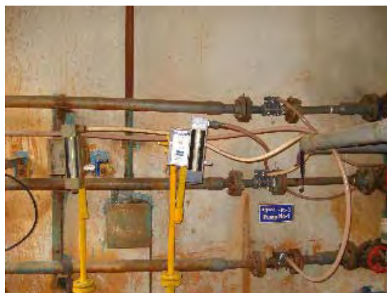
Figure3.13-5 Chlorine Dosage in Chandnighat Plant
