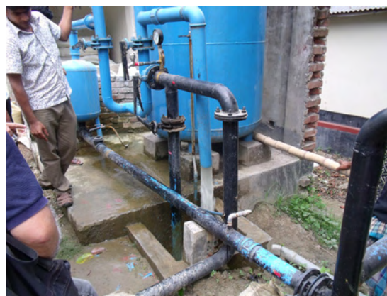
[Water supply facility in Fatenagar village of Keranjiganji district] Water source is groundwater. The tank is iron removal filtration facility.
