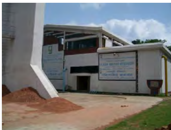
[Iron removal facility in Noakhali] The facility is constructed with the support of DANIDA. Iron is removed by oxidation with air diffuser and rapid sand filtration.
