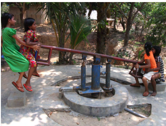
[Well with seesaw in a school in Lokkipur village of Gazipur district] It is an example of water supply and sanitation program by NGO and has 2 functions; to pump up from the well and to the elevated water tank.
