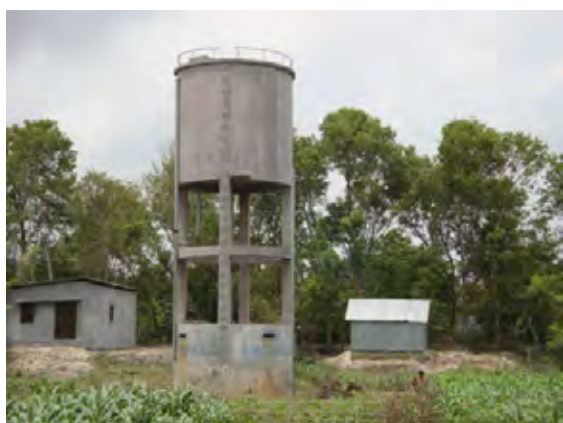
[Elevated water tank in Kachua village of Chandpur district] Groundwater is pumped up by well pump and distributed through the tower.
