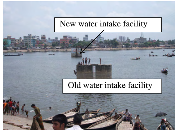
[Water intake facility Chandnigahd Purification Plant of Dhaka WASA] Water intake facility is 1km far from the plant. The old water intake facility is not used because of the decrease of water volume.
