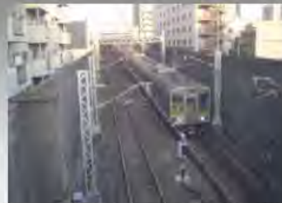
Water Stop High Retaining Wall
