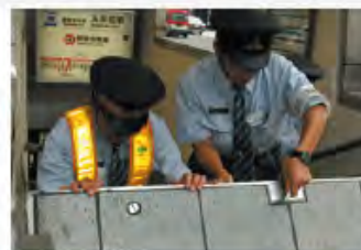
Installation for Water Stop
