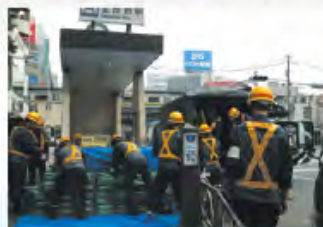
Installation for Water Stop
