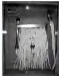
Distance of Hydrant in Station (25m)
