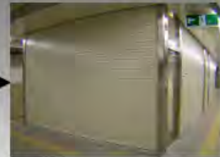
Fire Protection Compartment
