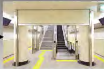
During Evacuation (Smoke Curtain)
