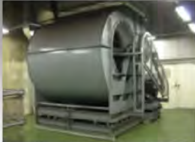
Centrifugal Tunnel Ventilation Fan Source: Rinkai Line, Japan
