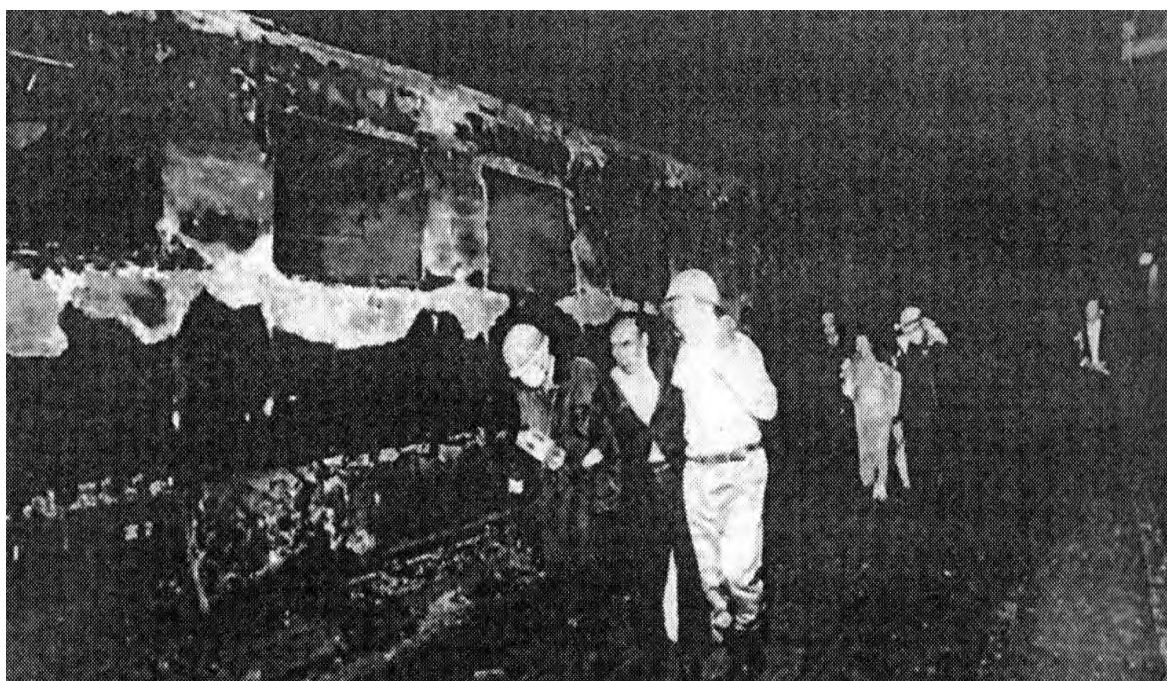
Figure 6-3 Picture at the Hokuriku Tunnel Fire Accident
