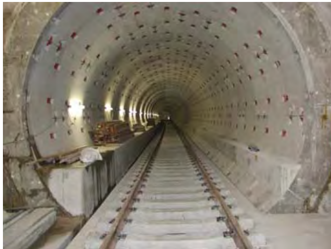
Figure 4-271 Resiliently-Supported Track
