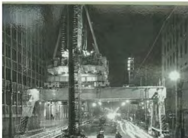
Figure 4-216 Special Equipment (Portal Frame) for Construction of Diaphragm Wall at Narrow Road
