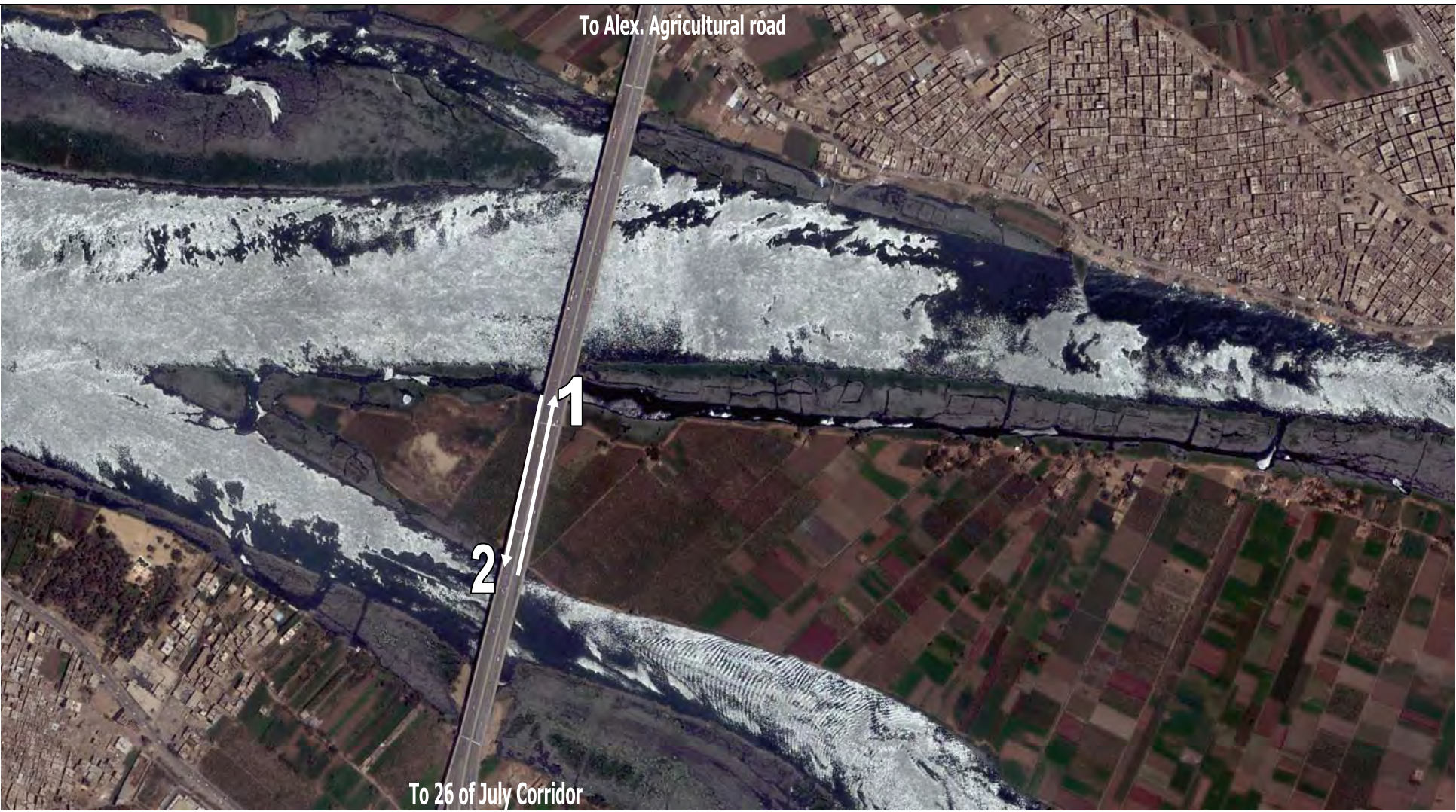
S9 - Ring road at Alwarraq bridge
