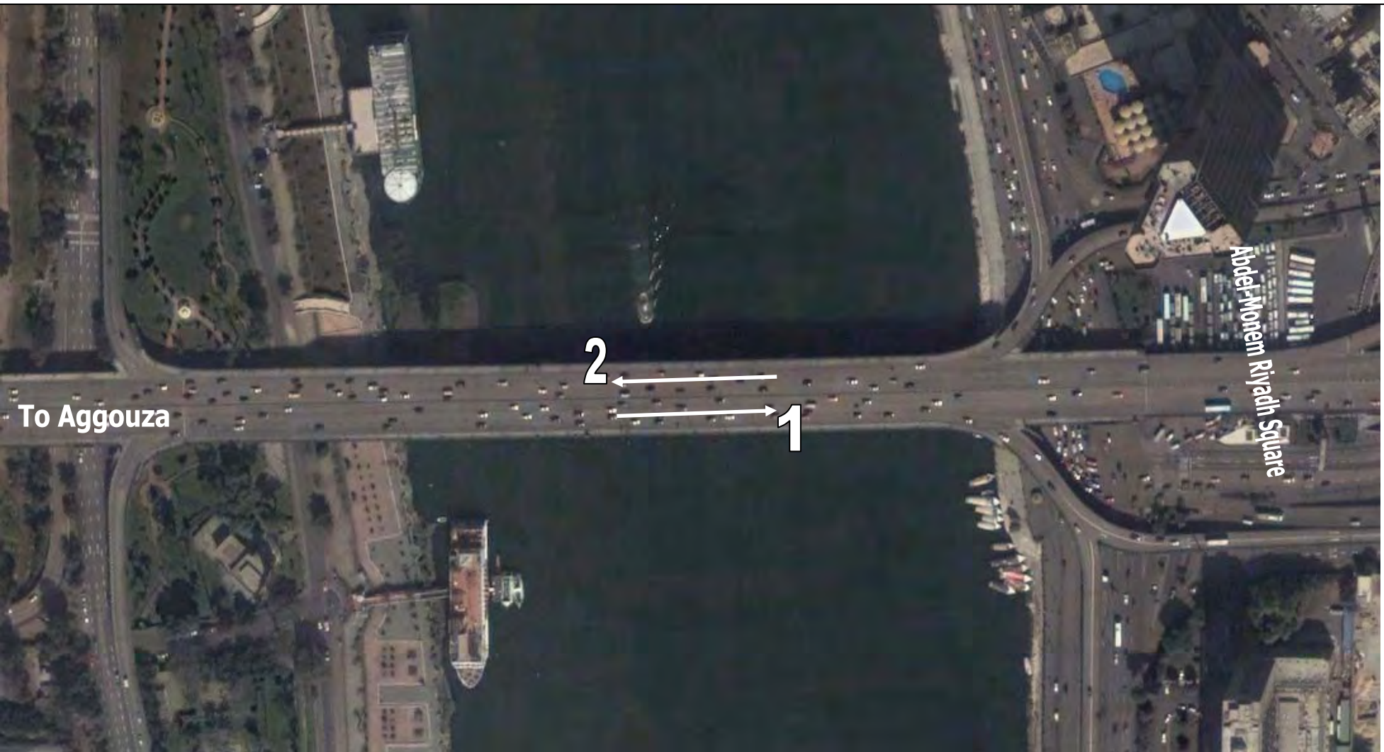
S5 – 6 of October bridge - between Abdel-Monem Riyadh Square and Zamalek ramps
