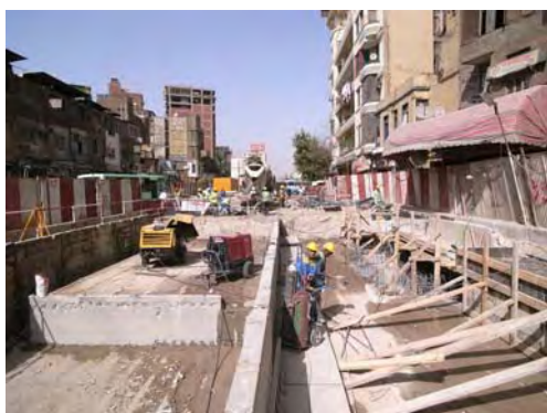
Figure 5-6 Cast in-situ Roof Slab of Underground Station
