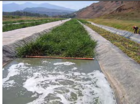
Bio-filter Treatment Plant of AMSA (April 4, 2006)
