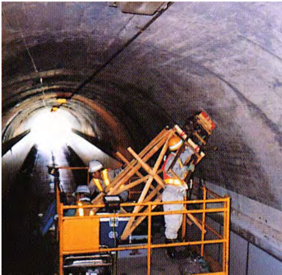
Chart 4.27 Inspection of occurrence of cavities behind lining by radar
