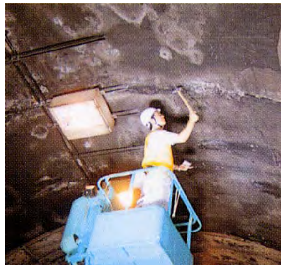
Chart 4.30 Inspection of condition of lining by hammerin
