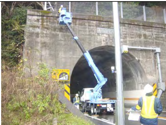
Chart 4.29 Inspection of occurrence of cracks by viewing
