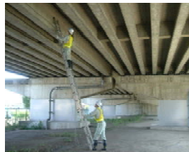
Chart 4.26 Scenes of inspection work for bridge
