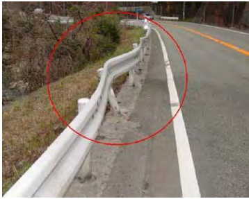
Damaged guardrail
