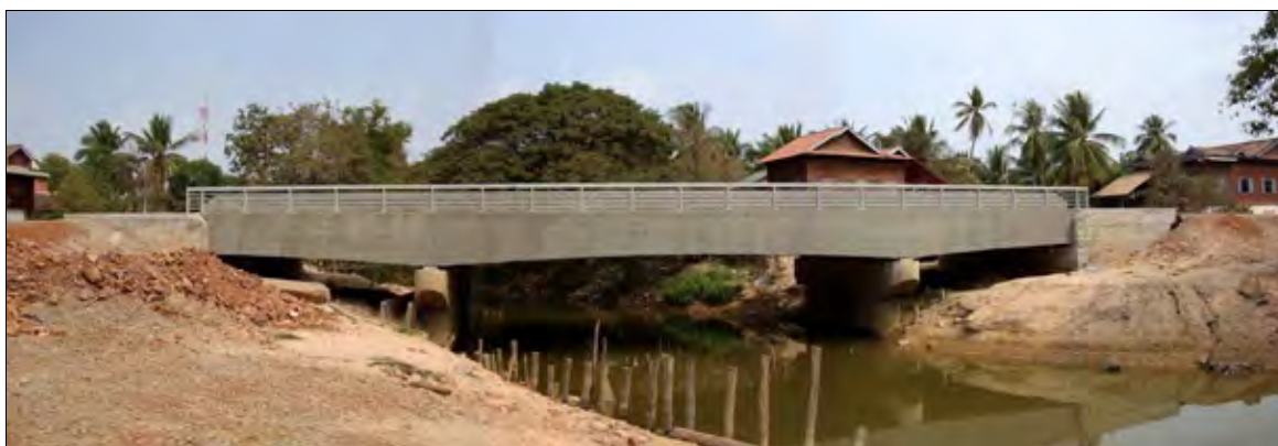
Photo 3-1 Side View of Ring Road Bridge over Siem Reap River
