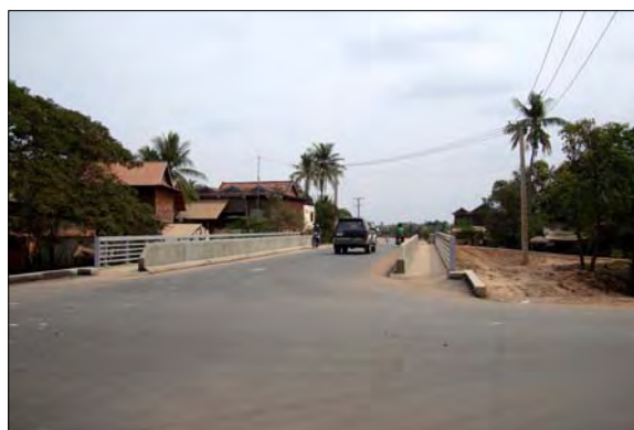
Photo 3-2 The bridge was opened to the public
