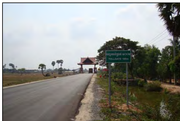
Photo 3-4 Tollgate and Tollgate Guide Sign
