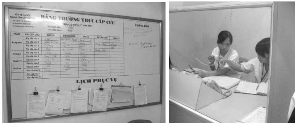
Figure 6.3.2 Center for Receiving of 115 Calls and Dispatching Ambulance Teams
