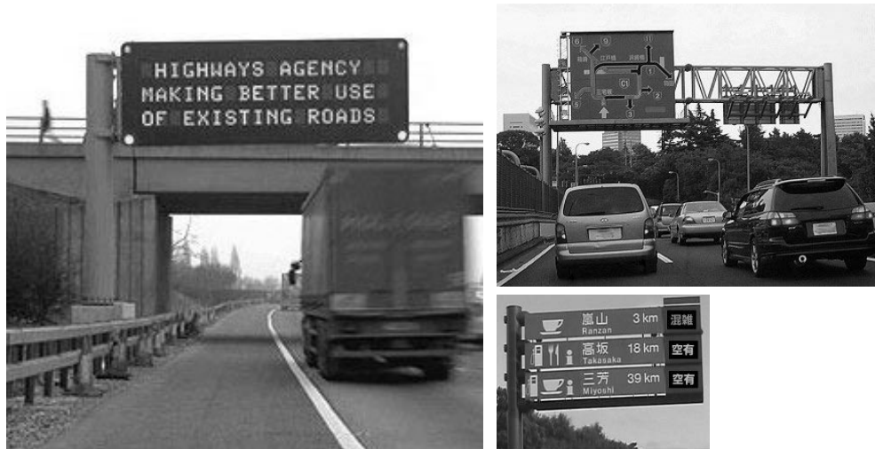
Figure 5.7.3 VMS/SGM on Roadside
