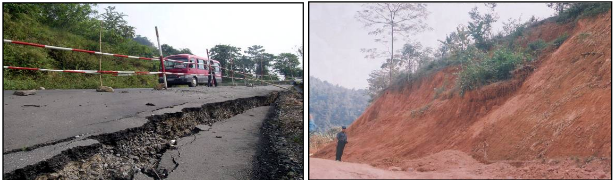
Landslide in Cao Bang Province
