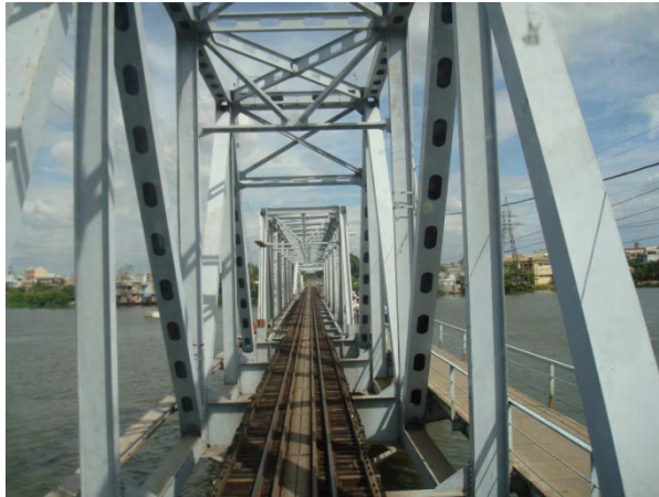
Figure 2.2.1 Truss Bridge with 1 Meter Gauge
