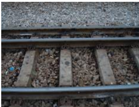
Figure 2.2.5 Concrete Sleepers and Vossloh Fastenings
