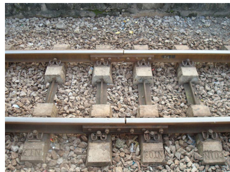
Figure 2.2.6 Suspending Joint
