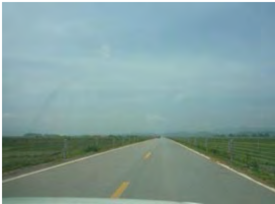
Photo-1 Condition of NH21
