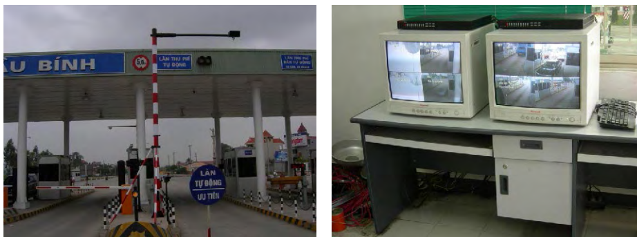
Figure 2.8.1 Toll Gate Lanes and Monitor Screen in Management Office
