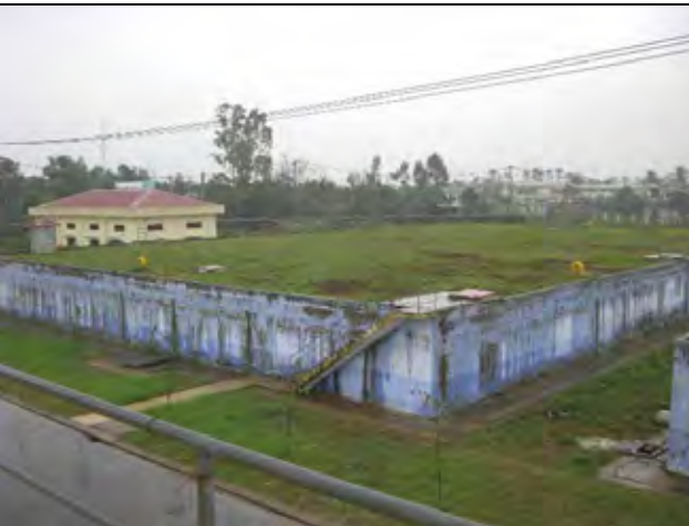
配水池(10,000m 3 ) x 2 (Cau Do 浄水場)
