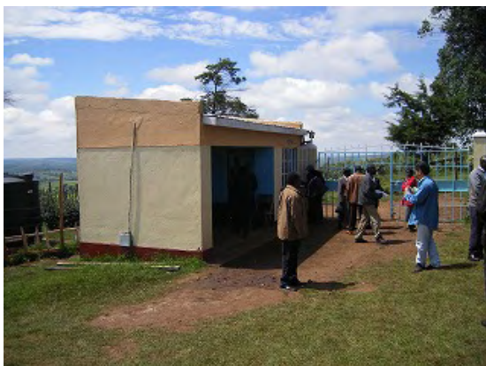
Security guards' room located next to entrance gate
