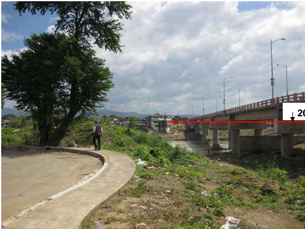
Photo-14 Tumana Bridge (downstream side view, Marikina River)
