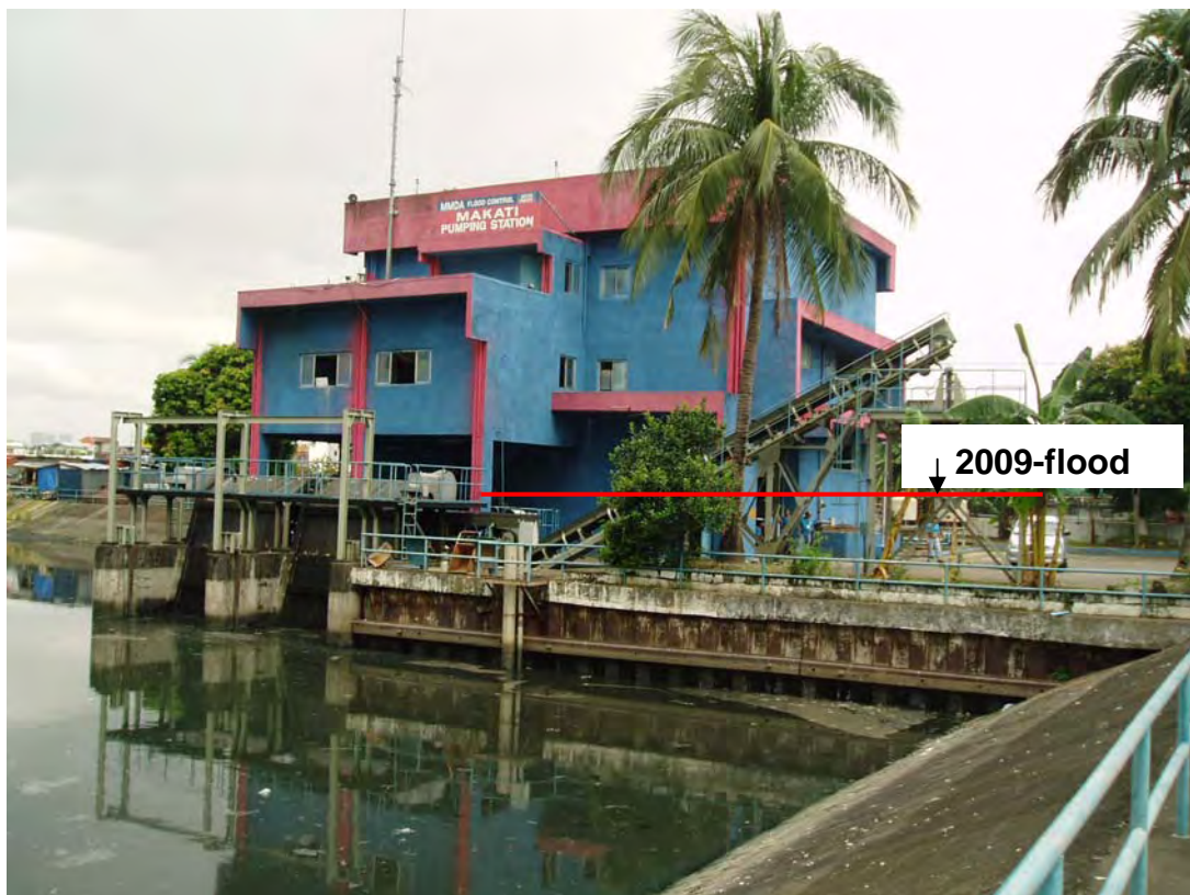
Photo-4 Makati Pumping Station (Metro Manila)
