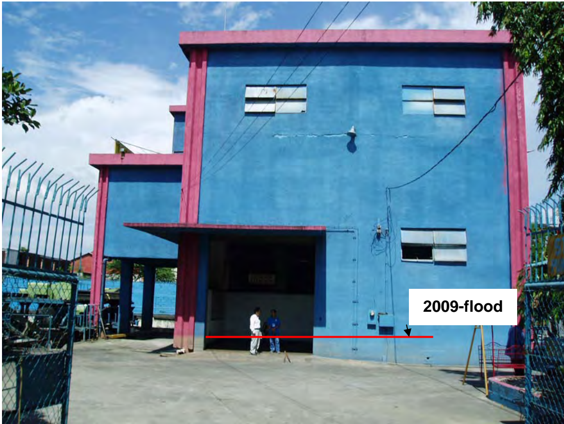
Photo-1 Sta. Clara Pumping Station (Metro Manila)
