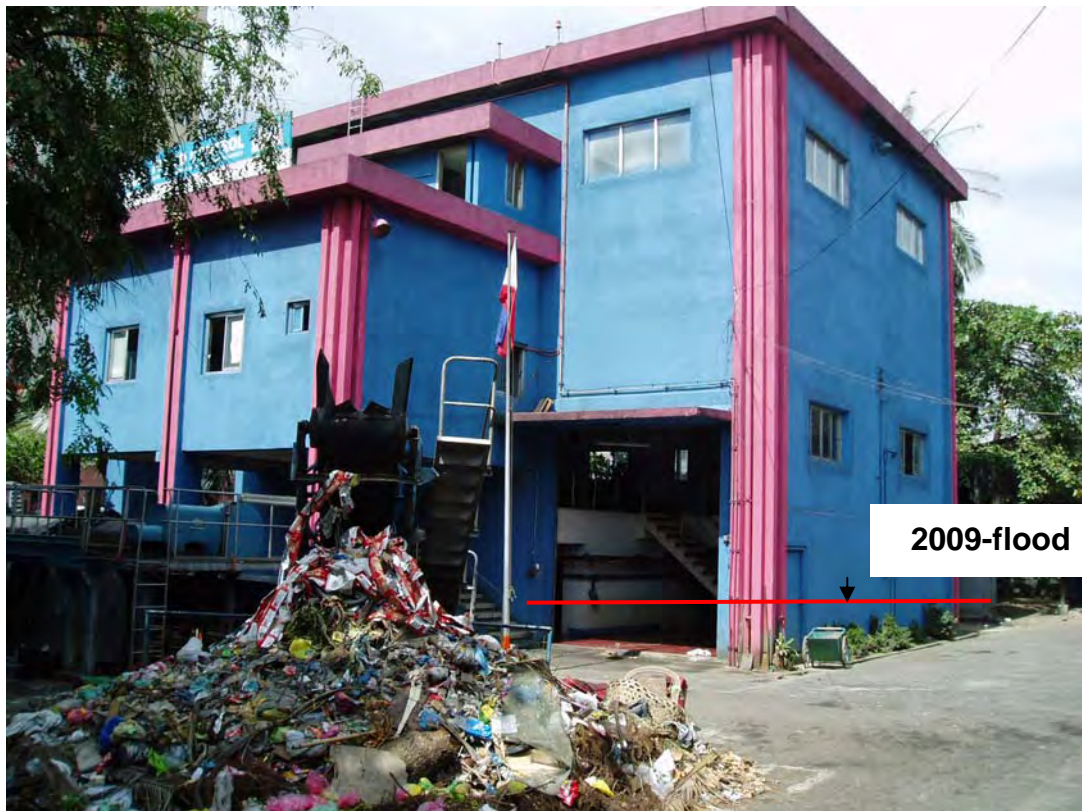
Photo-2 Pandacan Pumping Station (Metro Manila)
