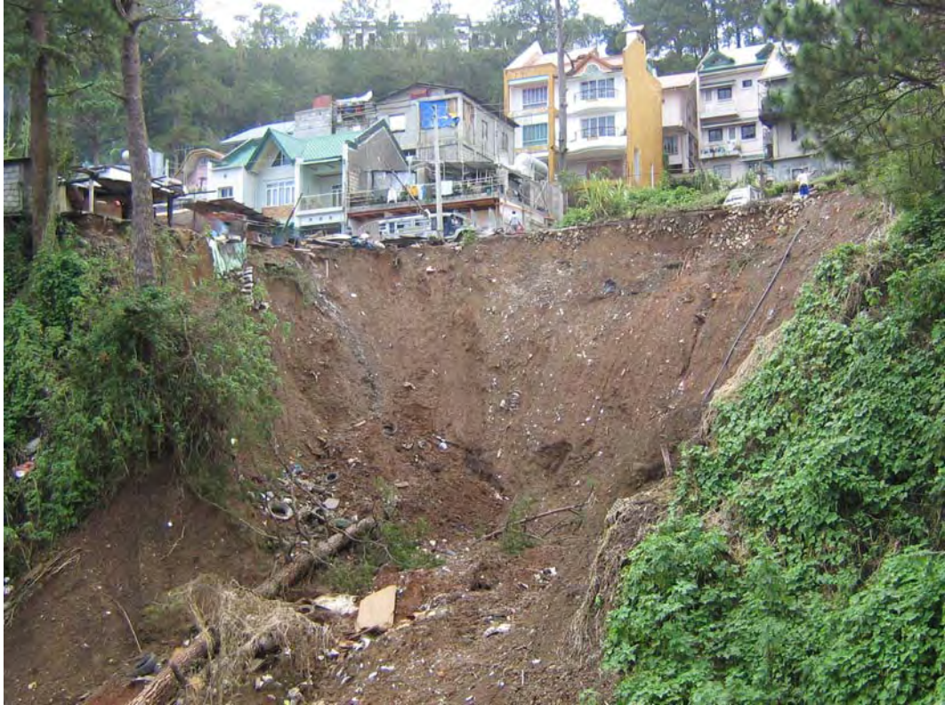
Photo-23 Landslide by Pepeng in United Residence Dominican Hill, Bgy. Upper Q. M. Baguio City (CAR Region)
