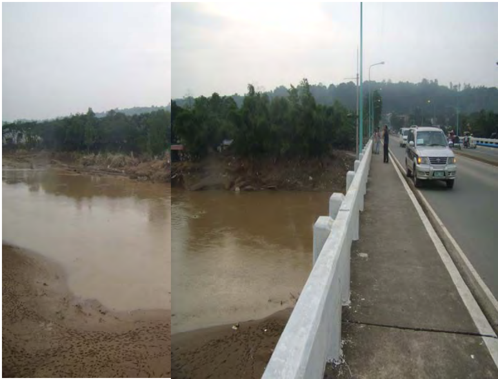
Photo-12 San Mateo Bridge (downstream view, Marikina River )
