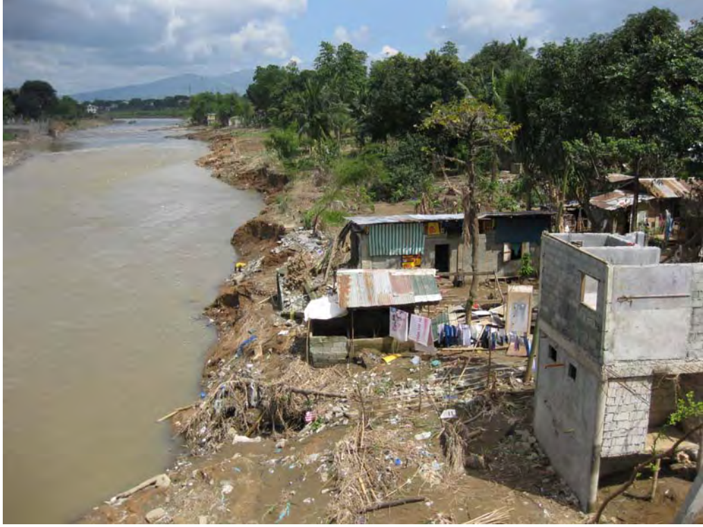
Photo-11 San Mateo Bridge (downstream view, Marikina River)
