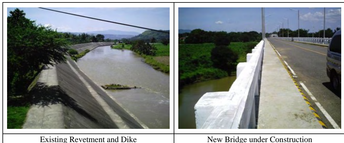
Figure R 6.2 Existing Dike along the River and Bridge under Construction
