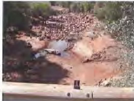
A dry river bed at Kapingazi water intake
