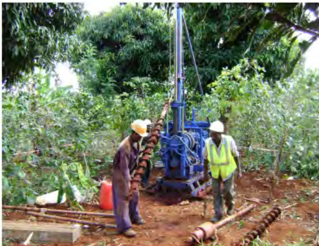
Plate No.3 : Drilling in Progress at Mukangu Water Treatment Plant
