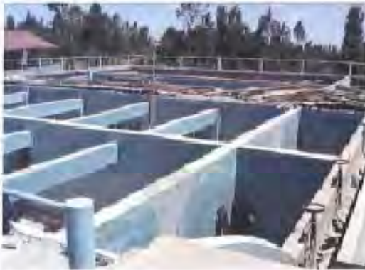
Mukangu water siltation tanks under repair
