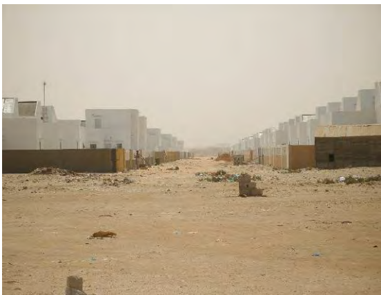
Figure 1.9 Residential district under construction
