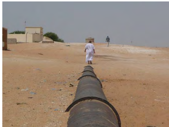
Figure 1.4 Main water pipe
