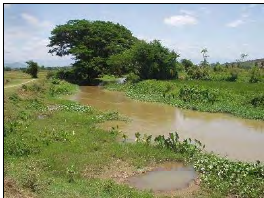
Water canal for rice irrigation. This type of canal is proposed to be the site for irrigation system construction. (Ninh Thuan province)
