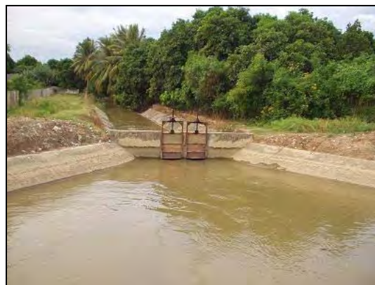
Cemented water canal and barrage for rice irrigation. This type of irrigation system will be constructed as “small scale infrastructure” (Ninh Thuan province)
