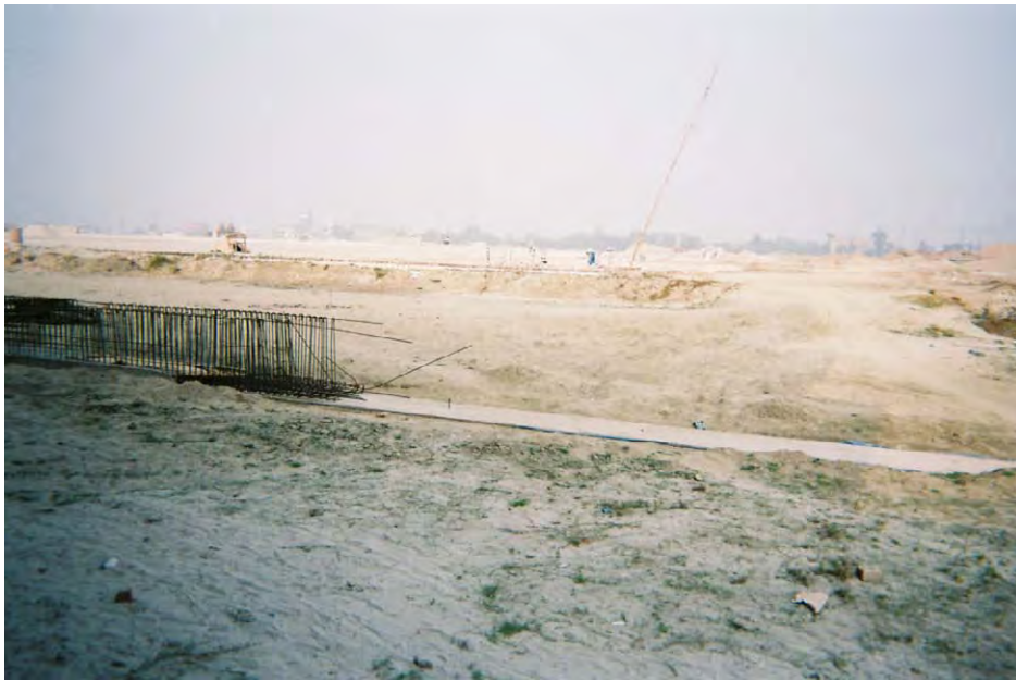
Photo 9.3-1 Pangaon( under construction)
