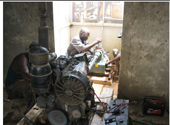
Small scale rehabilitation works
