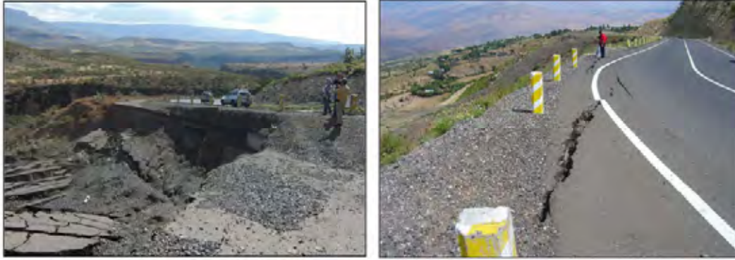
Figure 1-3 Points where Road Alignments Were Revised (left) and Points where Revisions of Road Alignments Will Be Needed (right)
