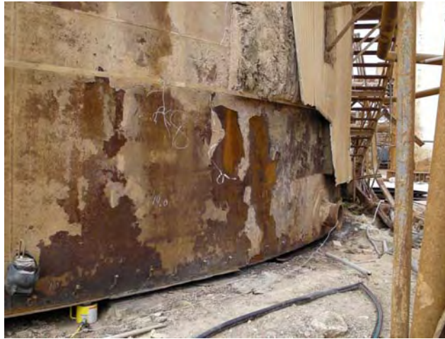
Figure 6.2-12: Current Condition of Sulfuric Acid Tank and Soil Condition
