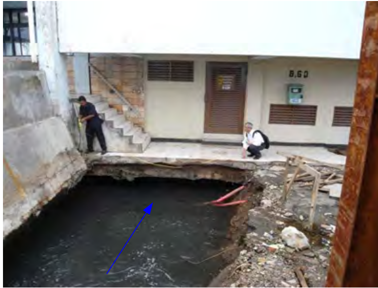
Photo-2.10 Inlet of Leakage flow under East Pump Station
