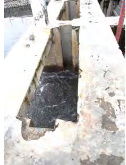
Photo-2.11 Blowout of Leakage Water in front of Pump No.1
