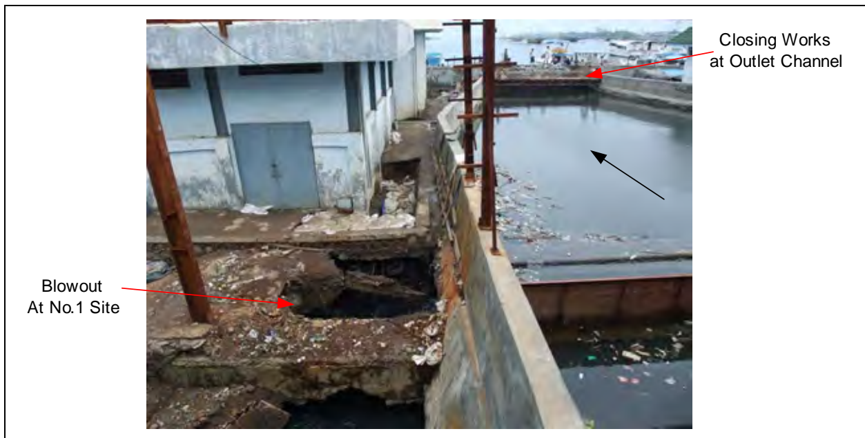
Photo-2.9 Situation of Piping Collapse at East Pump Station
