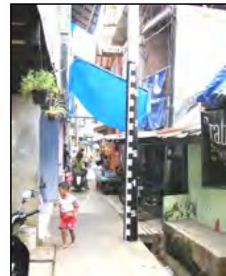
Staff Gauge installed in Kampung Melayu by JICA Project
