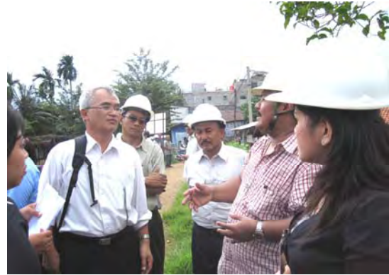
The Officer from BBWS Ciliwung-Cisadane and Contractor gave explanation about the design
