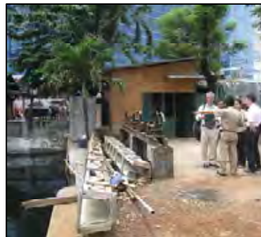
Gate Inspection to Jembatan Merah Gate (February 19 th , 2009)
