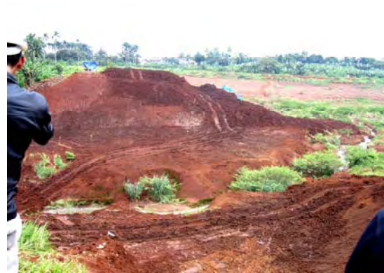
Condition of Situ Gintung when the visit conducted
