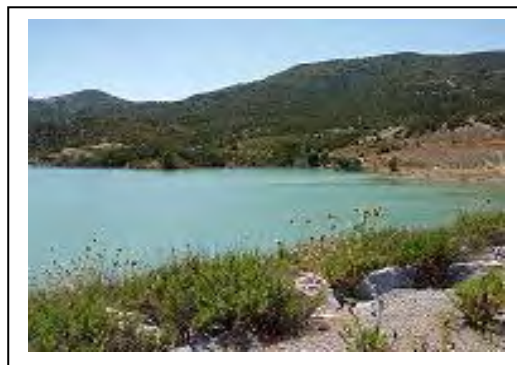
Kseub Hill Dam
