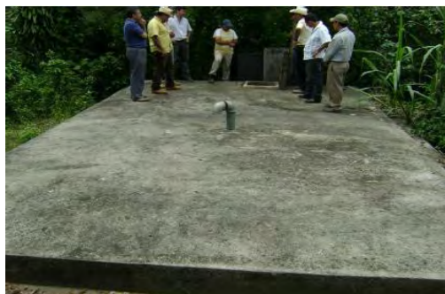
Water supply project in Bethel village
