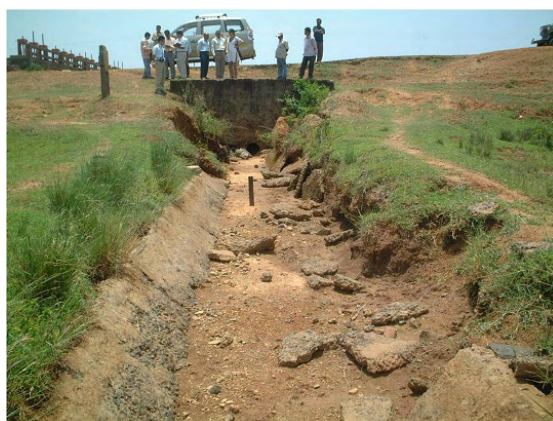
Fig. 6 Damaged Canal
