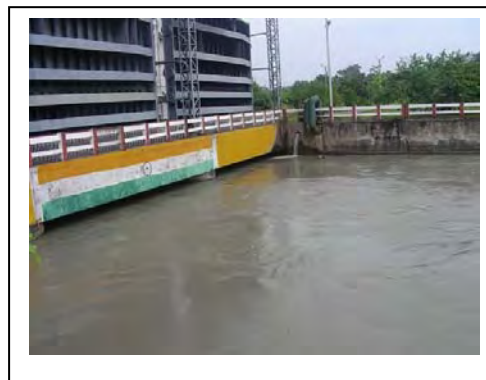
The power plant seen from downstream of the irrigation canal
