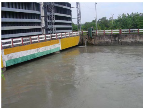
Fig. 1 Present Condition of the Outlet (One Generator Operating)
