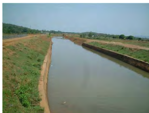
Main Canal developed by the Project
