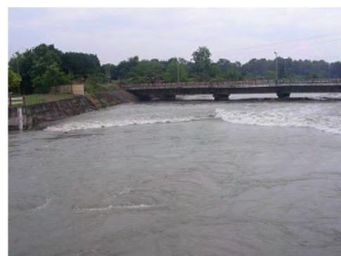
Fig. 2 Present Condition of the Outlet (Opposite Side)
