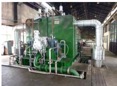
Figure 6: Gas Compressor after the Repair
