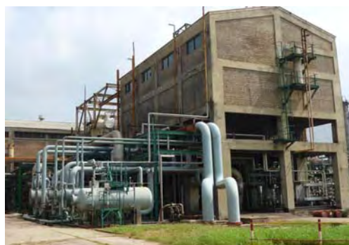
Figure 2: Ammonia Plant in the Fertilizer Factory
