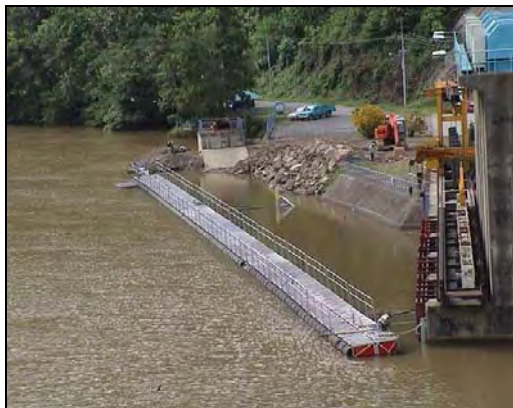
Photo 2: Water intake gate after the ex-post evaluation
