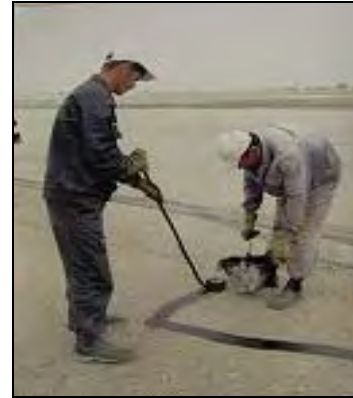
Photo 1 : Repairs with bitumen
