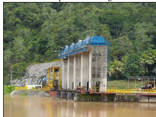
Photo 3: Water intake gate at the time of the ex-post monitoring
