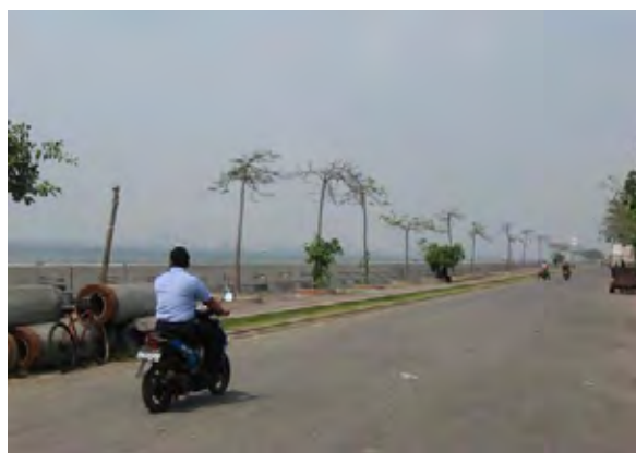
Completed east revetment water walls (July 2009)
