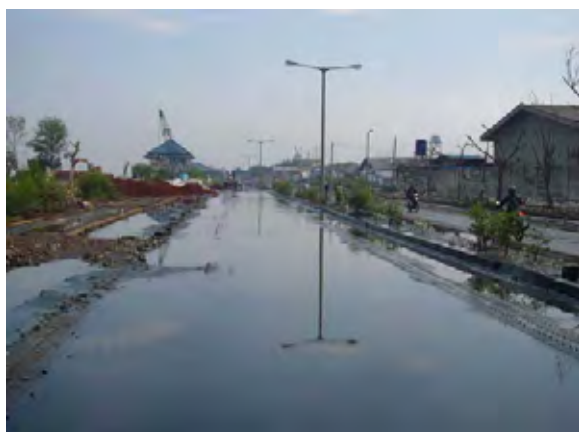
Flooding in JFP (May 2009)
