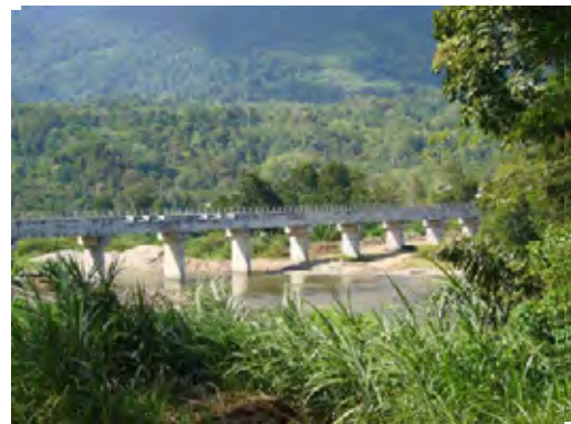
Batang Angkola Irrigation Aqueduct Bridge
