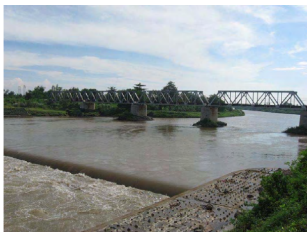
Groundsill down stream of a bridge in the Brantas River
