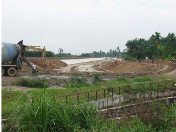
Link Canals under Construction in Ular
