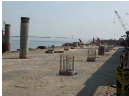
Pile foundation construction site
