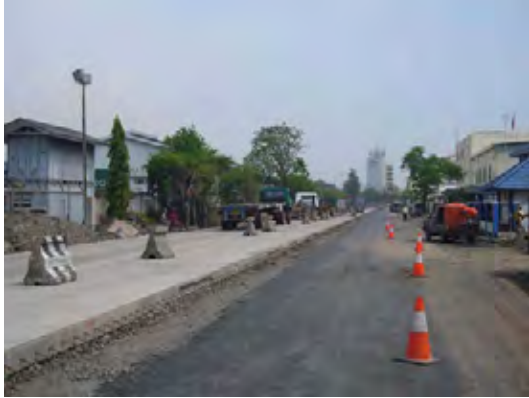
Improvement of port inner roads
