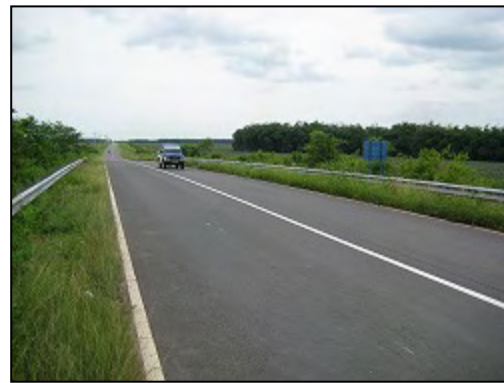
Project target road (Seputih Banyak – Manggala Section)
