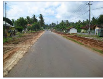
Ongoing road widening work (at the 2-3 km south from Jeparu)
