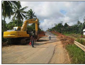
Ongoing road improvement work (at the 2-3 km south from Jeparu)
