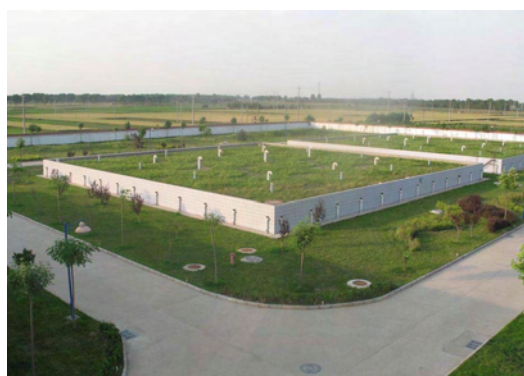
Water storage constructed by the Project in Luannan County
