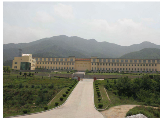
Yangjiadian Water Plant
