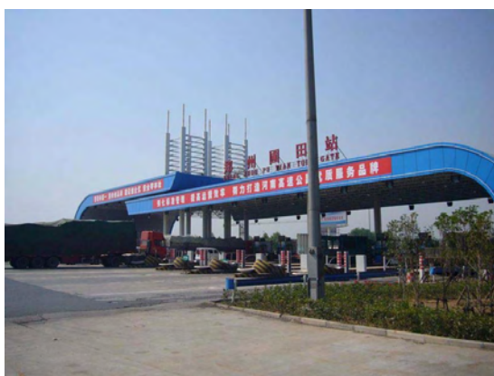
Toll stations at Putian Interchange
