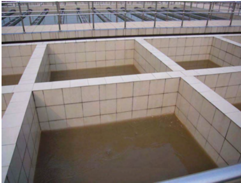
Settling tank of Fengshouba Plant
