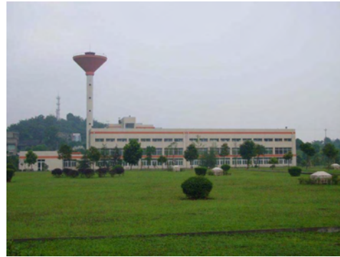
Fengshouba Water Plant Water Storage (Underground)
