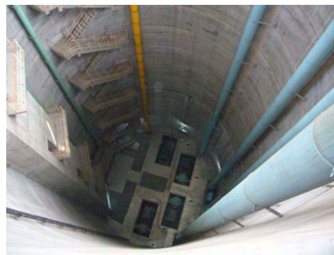
Receiving well of Fengshouba Plant
