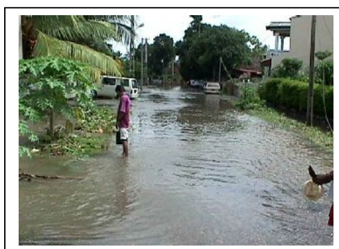
Flooding before the project (1998) (De Soysa road in Attidiya : phase III)
