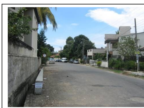
Inundation damages were reduced drastically after an underground drainage was constructed by the project (De Soysa road)
