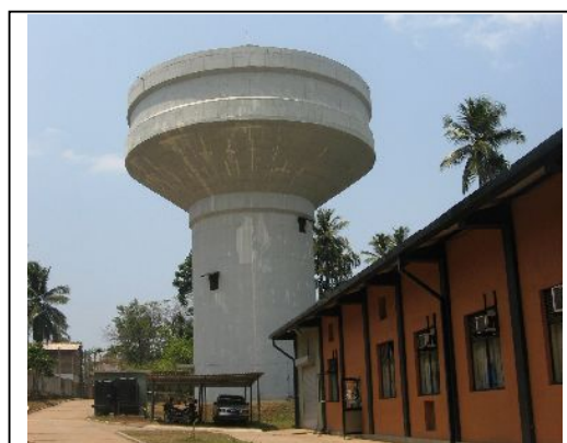
Tower and pump house in Mahara distribution center
