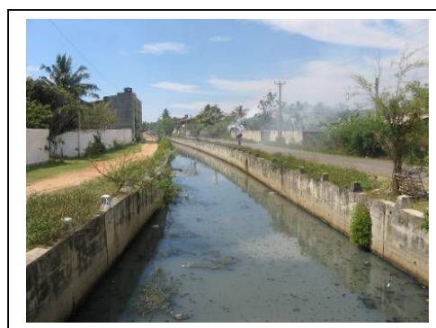
An improved drainage in Kaudana area
