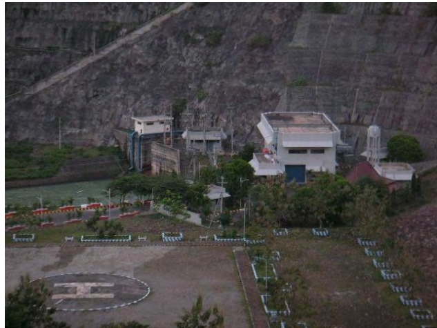
Distant view of Wonorejo Hydroelectric Power Plant
