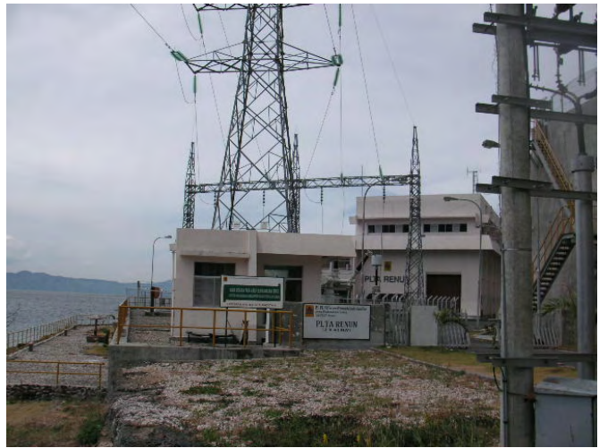
Renun Hydroelectric Power Plant Located at Lakeside Toba
