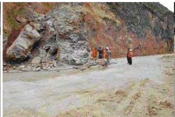
Removal of Fallen Boulder (Jauja-Tarma Highway)
