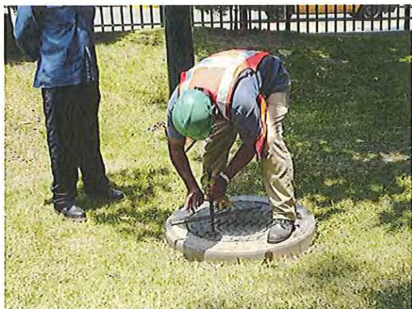
Manhole for the underground water distribution valve chamber at a public park
