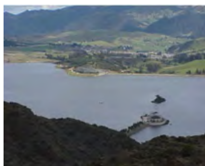
San Rafael Reservoir and Pumping Station
