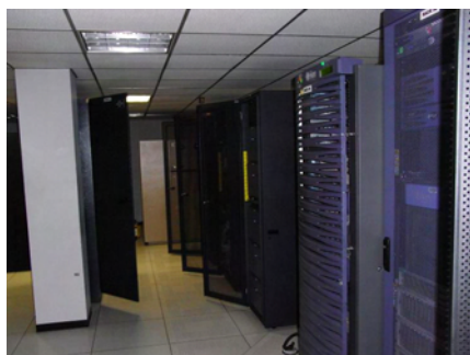
Figure 20: Computing system in the Control Center
