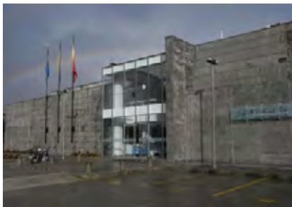
Figure 3: Outside View of Control Center
