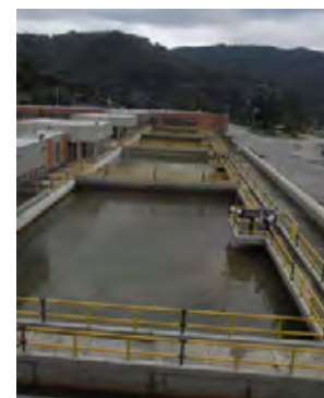
Figure 8: Wiesner Water Treatment Plant
