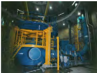
Figure 18: Pumping Station Facilities (the bottom floor)
