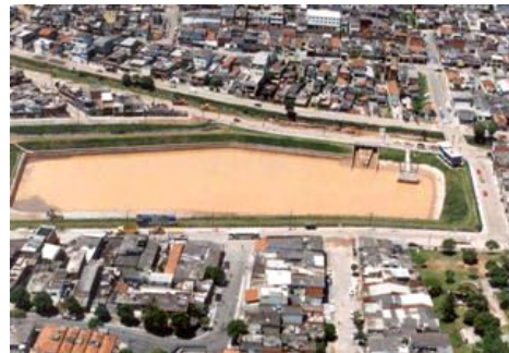
Figure 7: Rainwater Runoff Reduction Facilities (Flood Control Reservoirs)
