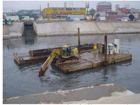
Figure 17: Work of Silt Removal
