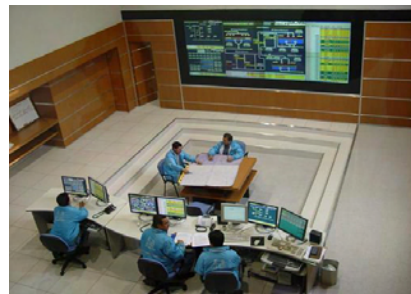
Figure 4: Control Room for Water Supply and Distribution
