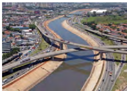
The Tietê River after River Improvement
