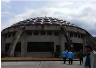
Figure 1: Outside View of Pumping Station
