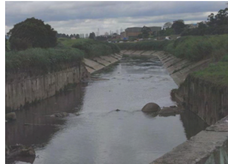
Figure 15: Cross-sections of the Cabuçu de Cima River. The near side is rectangular concrete, and the
