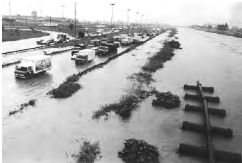
Figure 6 : Flood Damage in February 1983
