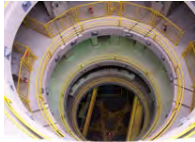
Figure 2: Inside View of Pumping Station (pumping units are set at the bottom)
