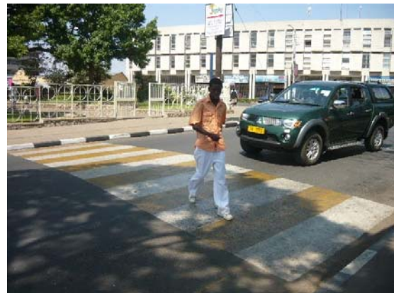
Photo 2.2-5 New type pedestrian Crossing This type has been adopted in Phase I with 3m width, therefore easy to see from driver seat
