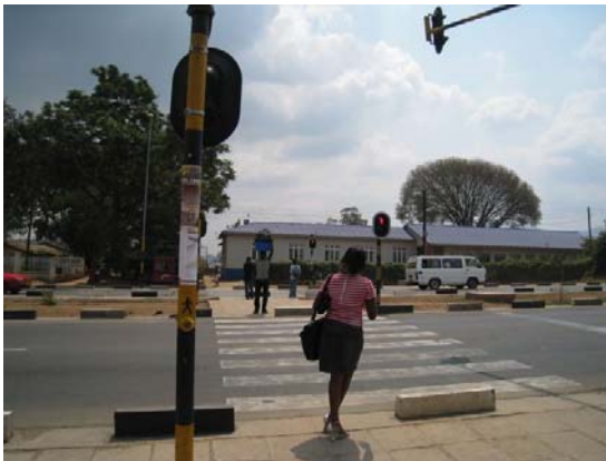
Photo 2.2-4 Ordinary Pedestrian Crossing Width is only 2m, therefore difficult to see from driver seat
