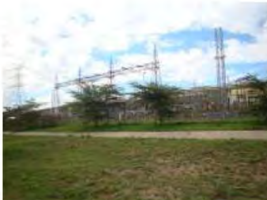
Olkaria Power Station II Near Olkaria Gate, Hell's Gate N.P.
