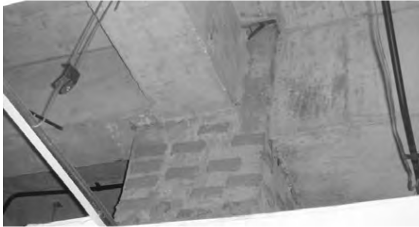
Photo of repaired column at Floor-3.
