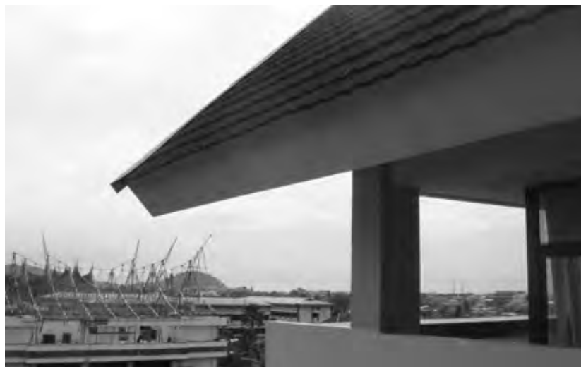
Roof of BPKP Building
