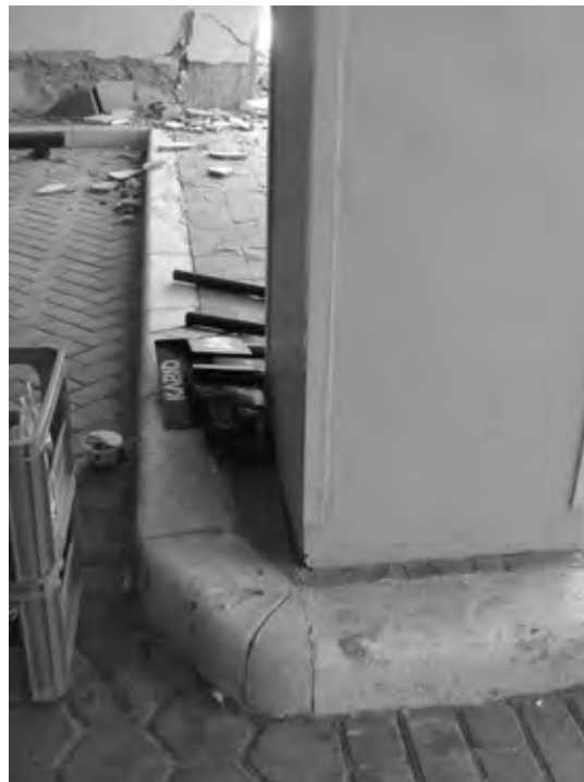
Photo of Column at Floor-G
