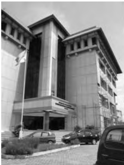
Figure 3.2.13 Outdoor View of UNP Building
