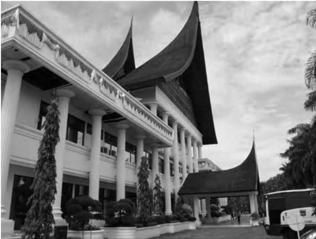
Figure 3.2.22 Outdoor View of the DPRD Building
