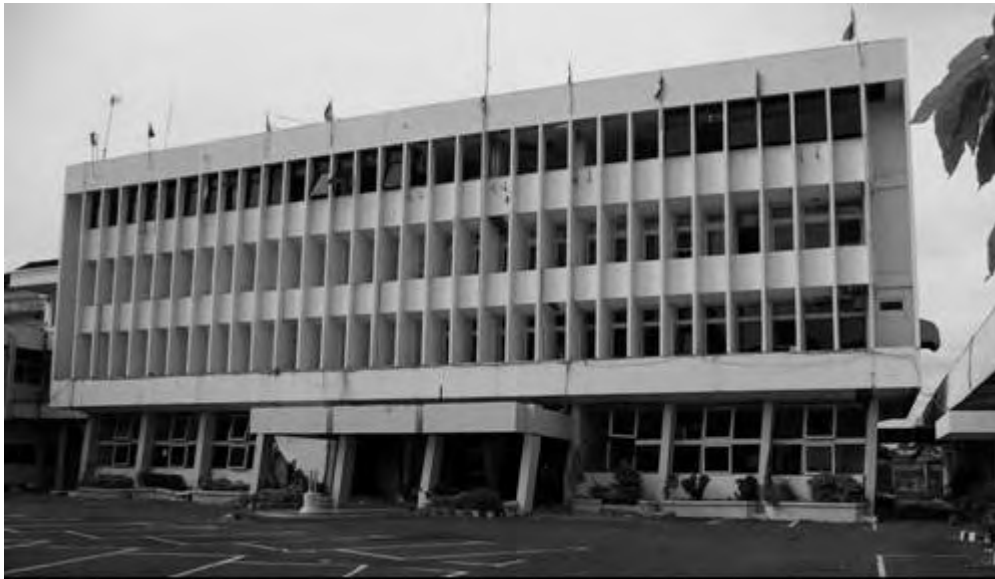
Figure 3.2.10 Exterior Appearance of PU Building
