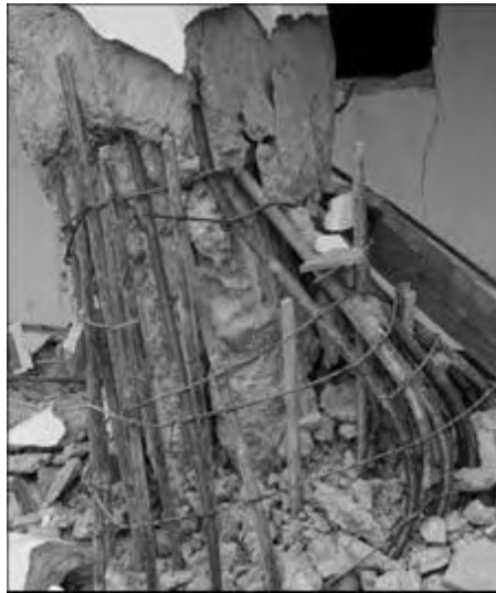
Figure 3.5.6 Detachment of tie hoop head
