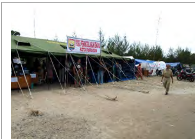
POSKO at Kota Pariaman. The Office Building in Kota was damaged and no longer usable. Temporary accommodation had to be established in front of the building
