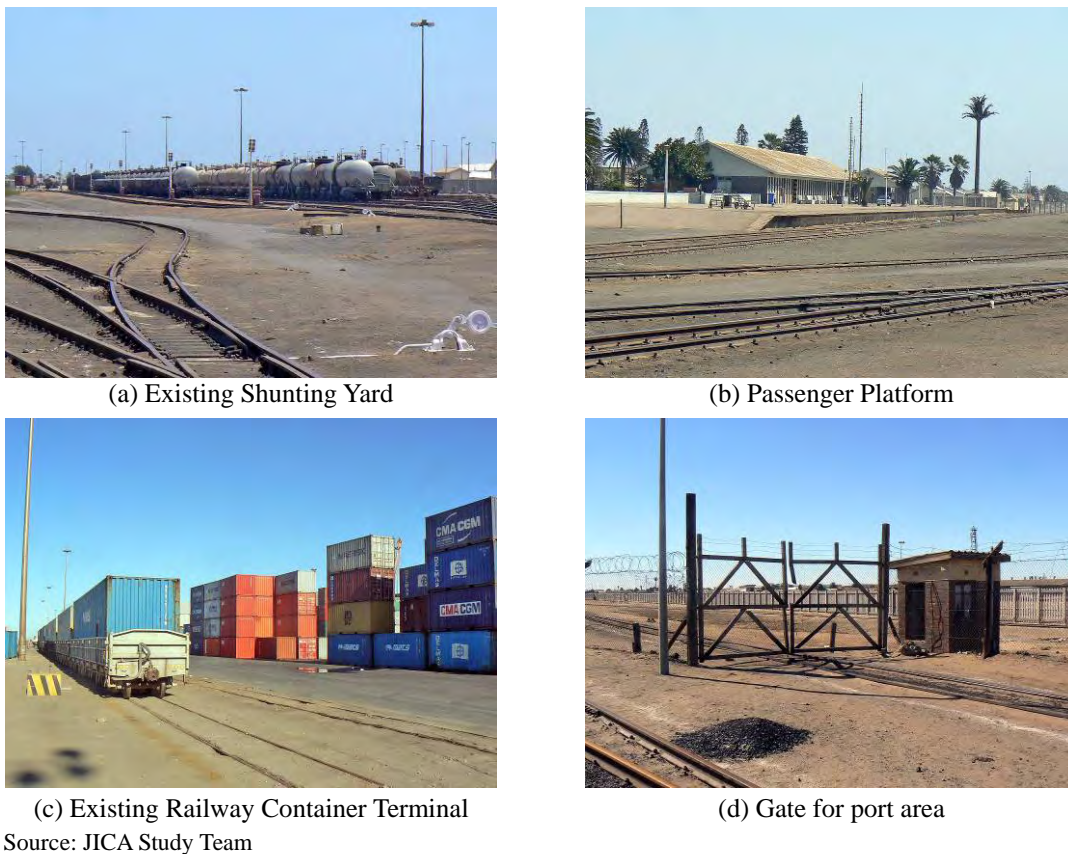
Figure 4.2.5 Photos of Existing Railway Yard in Walvis Bay
