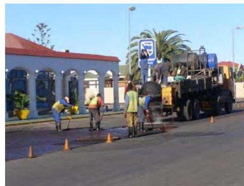
Asphalt paving works in Walvis Bay
