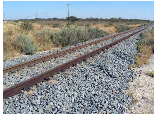
(b) 48 kg/m Rail with PC Sleeper
