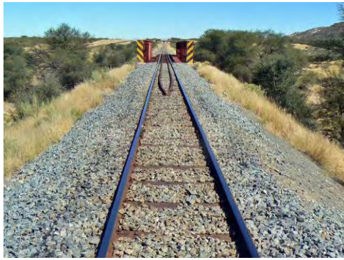
(a) 30 kg/m Rail with Steel Sleeper
