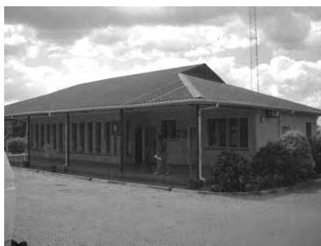
Photo-1 Border post main office
