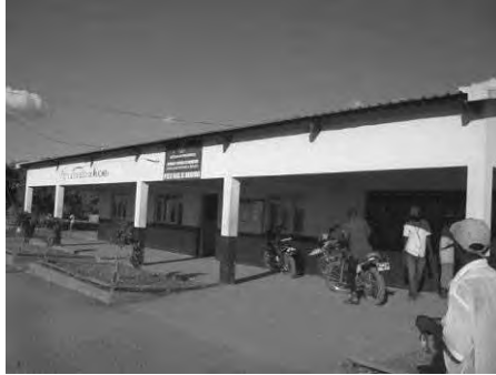
Photo-1 Border post main office
