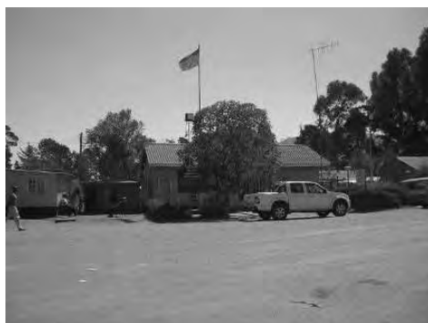
Photo-1 Border post main office
