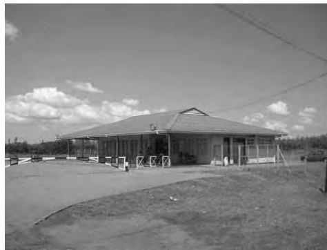
Photo-1 Border post main office
