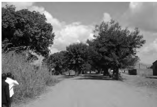
Photo 1.2.3 Road Lined with Trees (149km)
