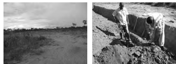
Photo2.1.4 B.P.7 (Borrow pit)
