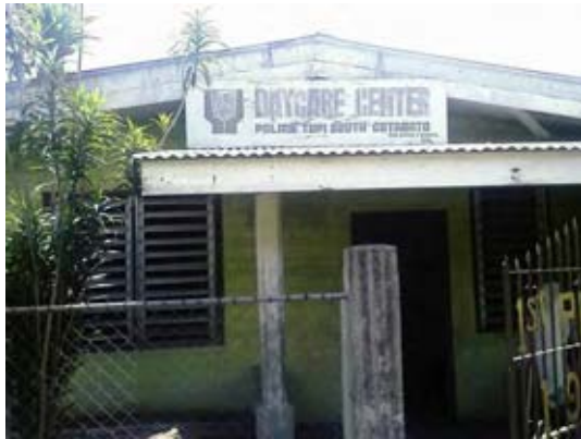
Figure O3.1-37 Exterior view
