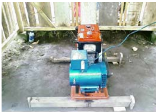
Figure O3.1-3 Generator
