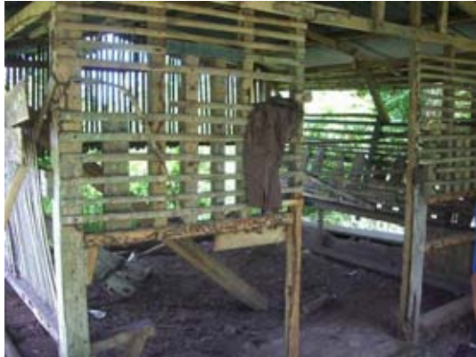
Figure O3.1-1 Old shed of generator
