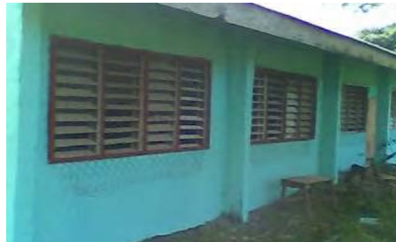
Figure O3.1-44 Exterior view 2
