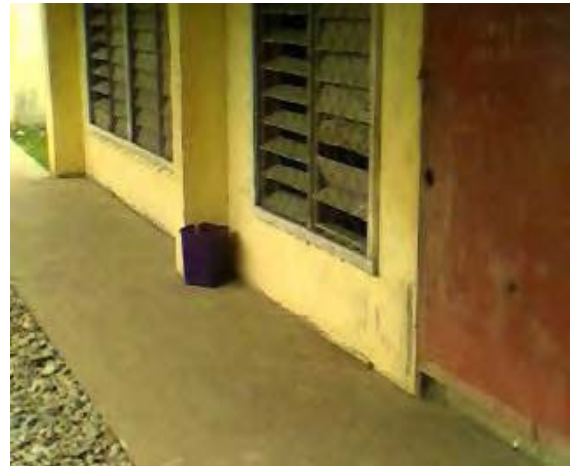
Figure O3.1-42 Exterior view 2
