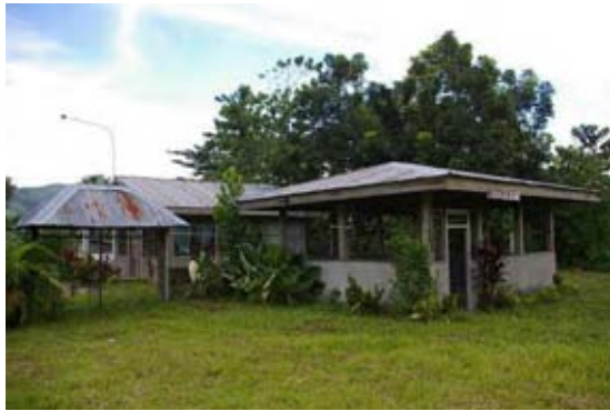
Figure O3.1-33 Exterior view
