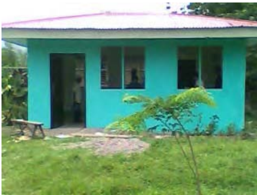
Figure O3.1-35 Exterior view
