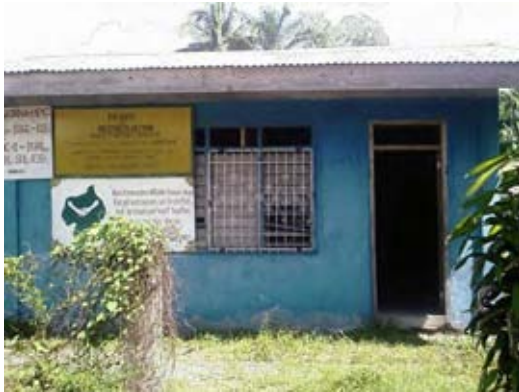
Figure O3.1-25 Exterior view
