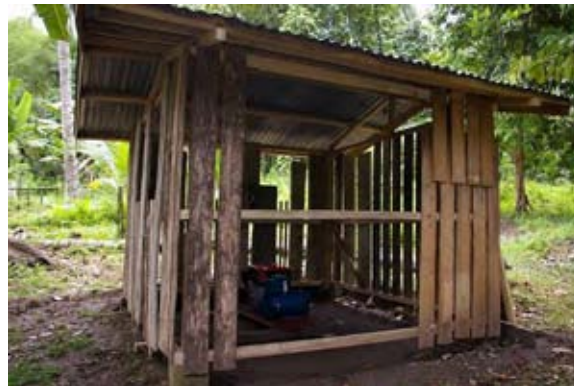
Figure O3.1-4 Shed of the generator
