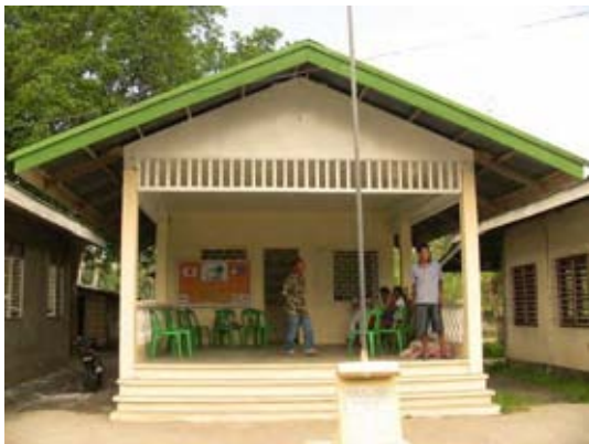
Figure O3.1-31 Exterior view
