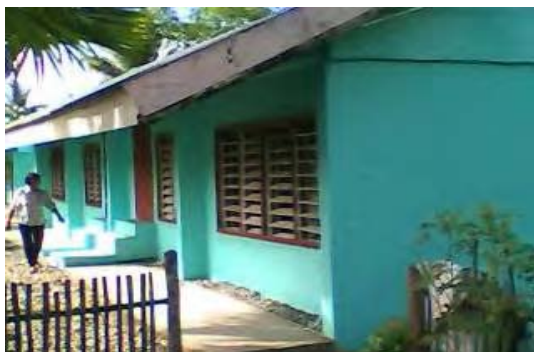
Figure O3.1-43 Exterior view 1
