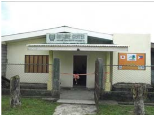
Figure O3.1-39 Exterior view
