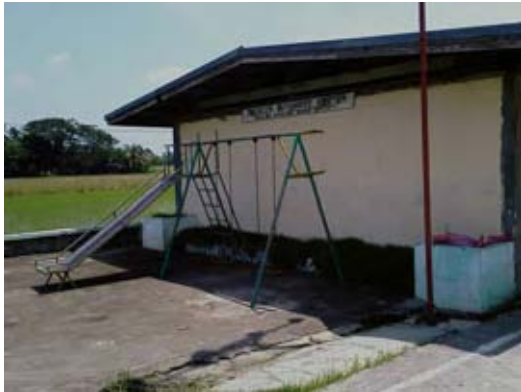
Figure O3.1-21 Exterior view
