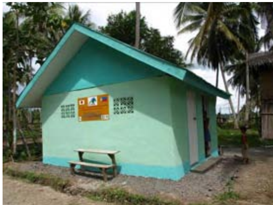
Figure O3.1-20 Comfort Room
