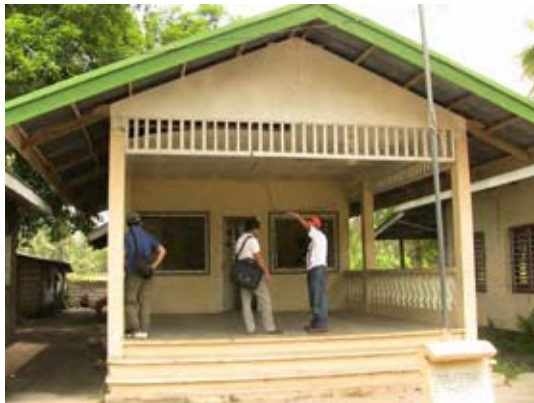
Figure O3.1-29 Exterior view
