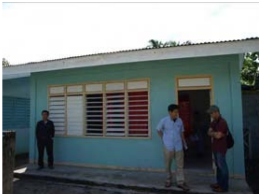
Figure O3.1-27 Exterior view
