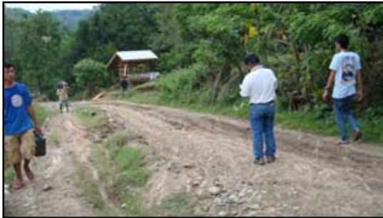
The existing road to be rehabilitated part of the bridge approaches
